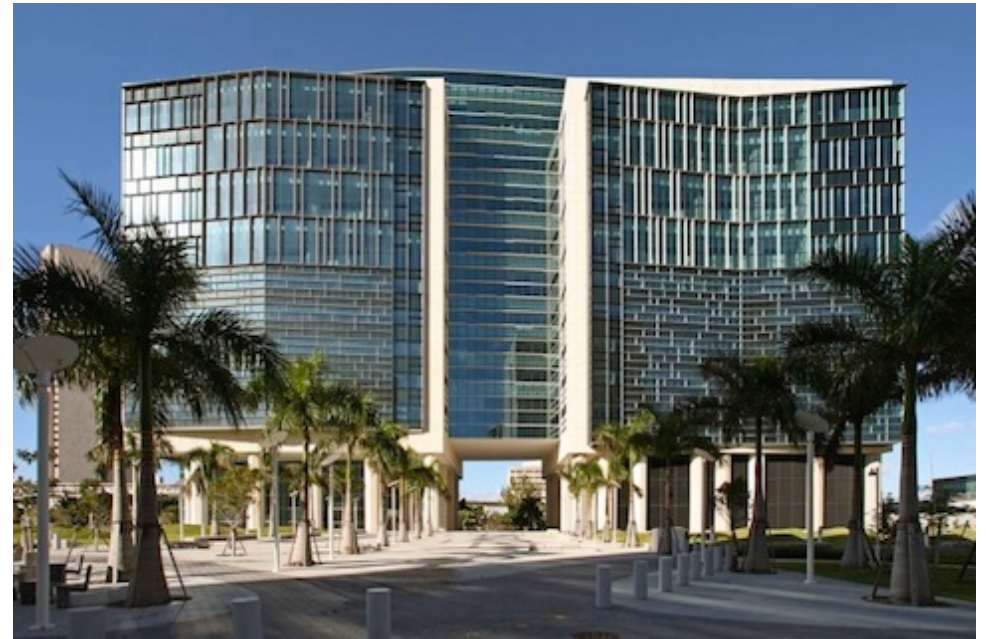
Ferguson Courthouse in Miami: Built in 2007
