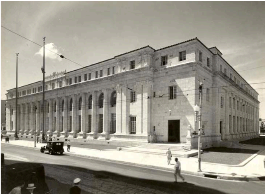
Dyer Courthouse in Miami: Built in 1931 Architect: Phineas Paist
